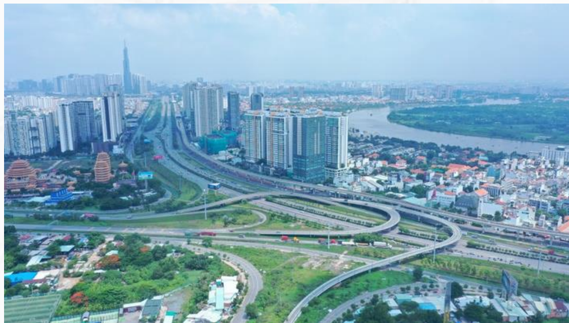
HANOI HIGHWAY EXPANSION PROJECT
