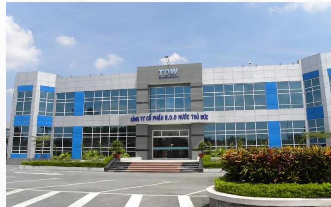
THU DUC B.O.O WATER PLANT
