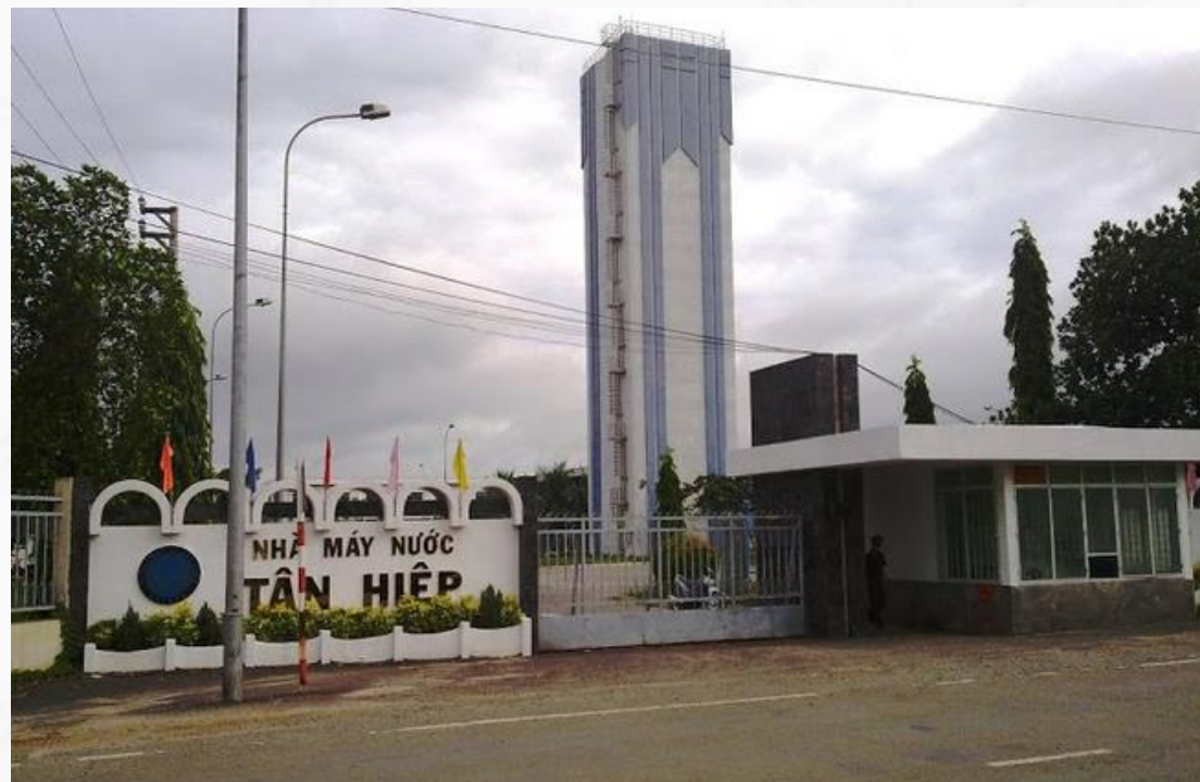
TAN HIEP 2 WATER PLANT
